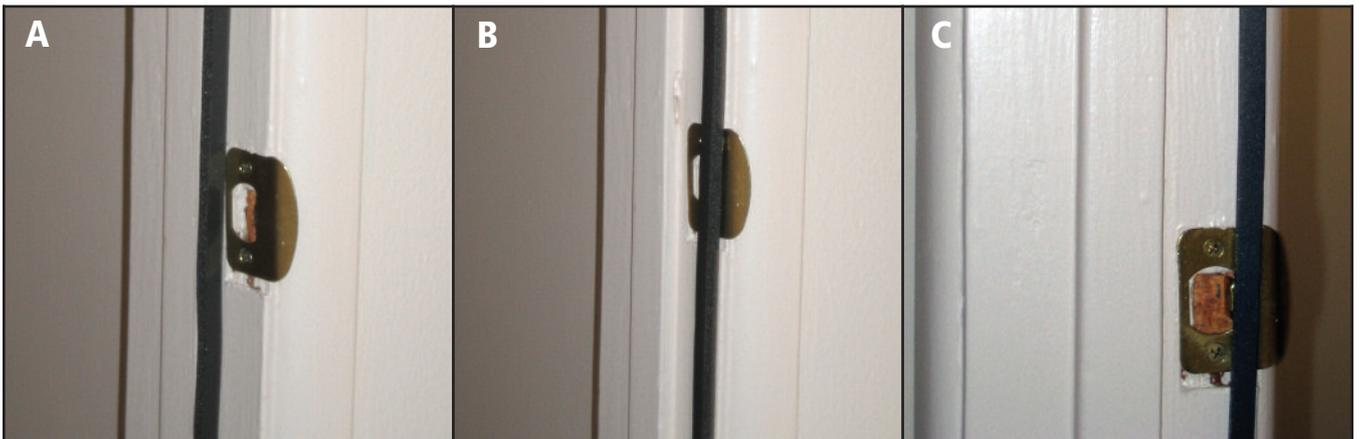
**Figure 7.** Install gasketing so that it's compressed by the door when you close it (A). Don't put it along the edge where the striker plate goes (B and C); it may seal tightly at first, but as you use the door, friction will cause it to eventually get torn loose.
