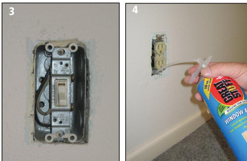
Figure 3. The air gaps and holes around fixtures like this light switch all leak sound. Seal them!
